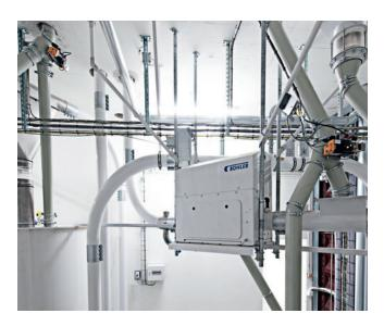
Flexible, product-friendly, hygienic, and safe – this and much more characterizes our pushing elements TUBO LBGA. Energy requirements are massively reduced in comparison with pneumatic conveyor systems and the layout can be extremely flexible.
